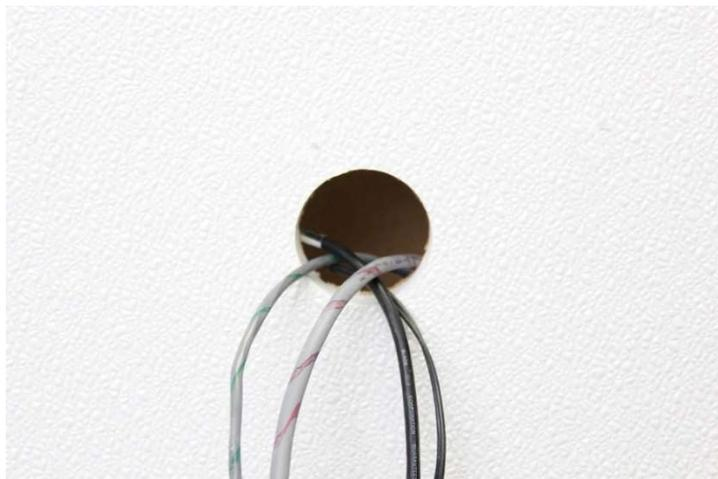
**Figure 7 - Hole for TIU Wiring**
